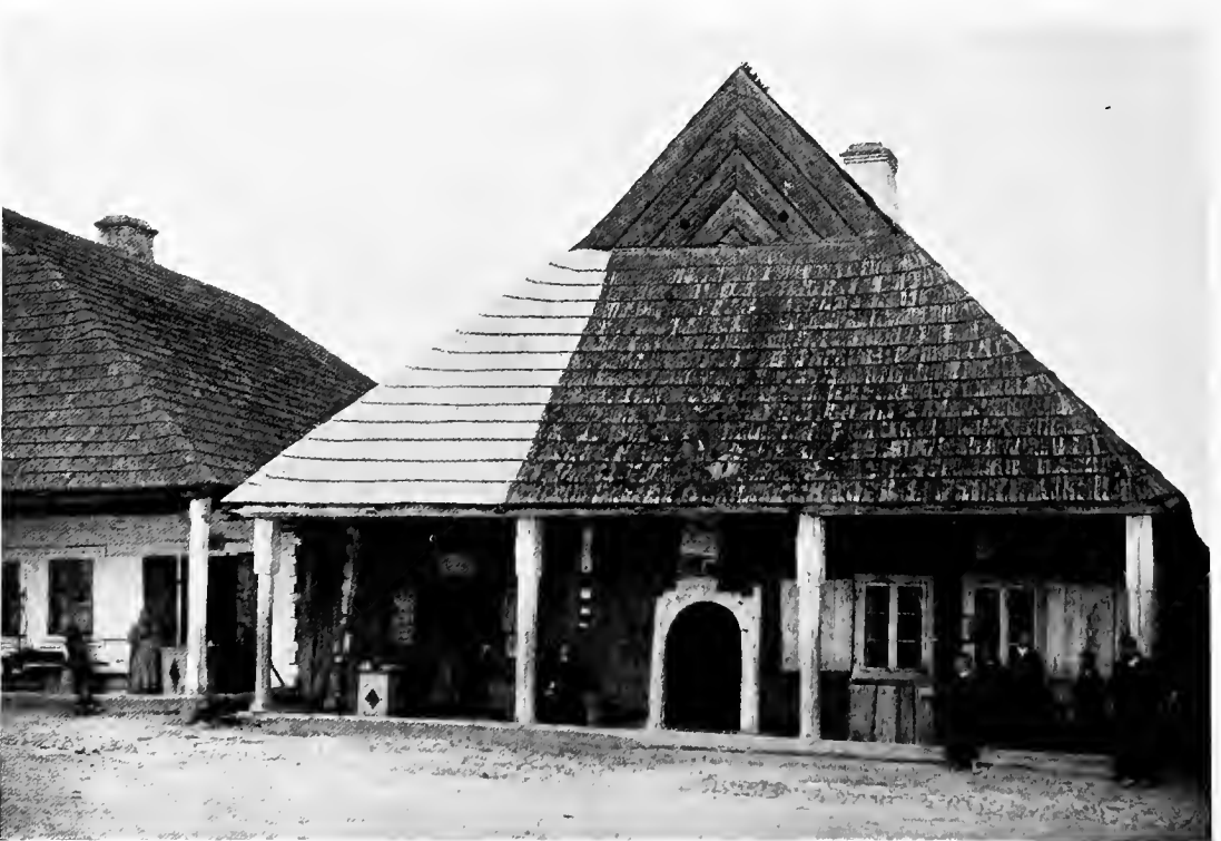
499 PEASANT'S HOUSE IN URZĘDOW
